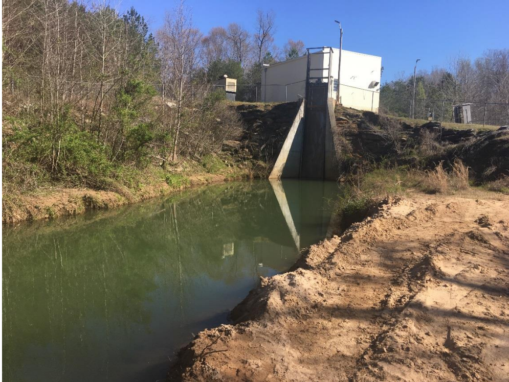
First Broad River Intake and Raw Water Pump Station
