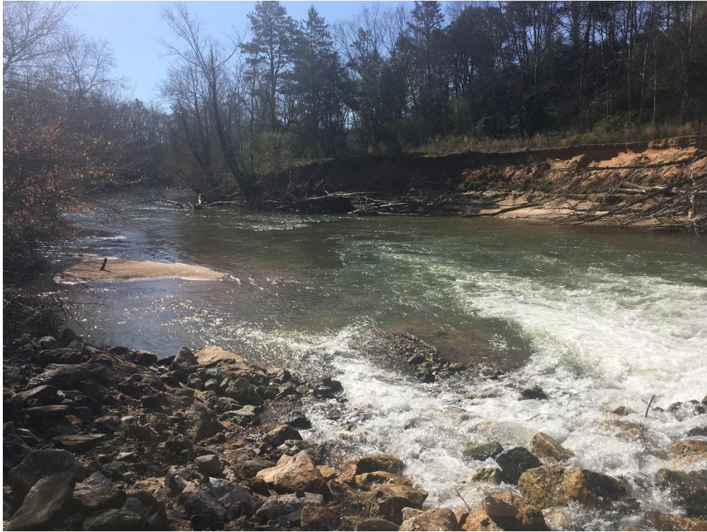
Bank Erosion Downstream of Weir
